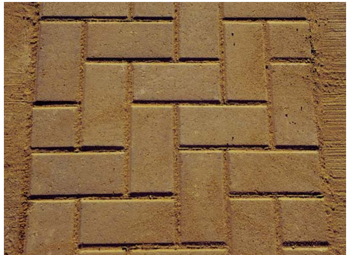
Figure 2. Chamfers on concrete pavers offer water drainage, increasing skid resistance and can decrease vehicle stopping distances.
