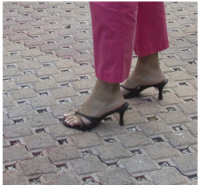
Figures 6 and 7 demonstrate permeable interlocking concrete pavement passing two important tests. The pavement passed the water infiltration test when water from the truck immediately disappeared into the surface. Just a few days prior to this test the parking lot took in a 3 in. (75 mm) rain storm with no runoff. The pavement also passed the high heel test demonstrating compatibility between fashion and environmental responsibility.
