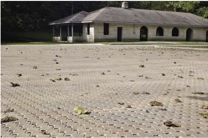
Figure 1. The permeable pavement eliminated the need for detention ponds that wouldn't fit on the site if conventional impervious pavement was used. Once a WPA project, the renovated picnic shelter make it easier to enjoy the huge trees, creek and waterfalls in the park.
