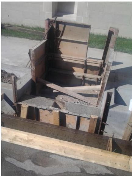
Constructing the tree planters. Curb turn-ins divert water to the trees.
