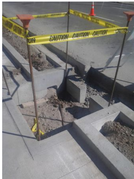
Constructing the tree planters. Curb turn-ins divert water to the trees.
