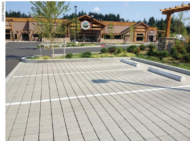
Permeable paver lot in front of Chuck’s Produce
