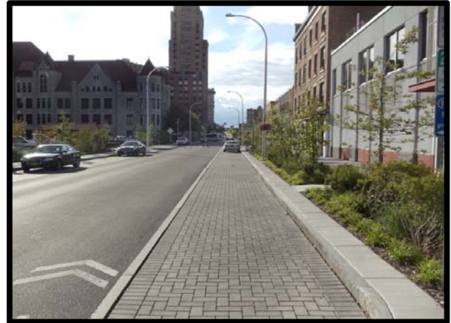
Urban Street After with Porous Paver parking Lanes and Bioretention, Syracuse, NY
