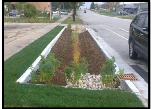
Terrace Bioretention Installation, Milwaukee, WI
