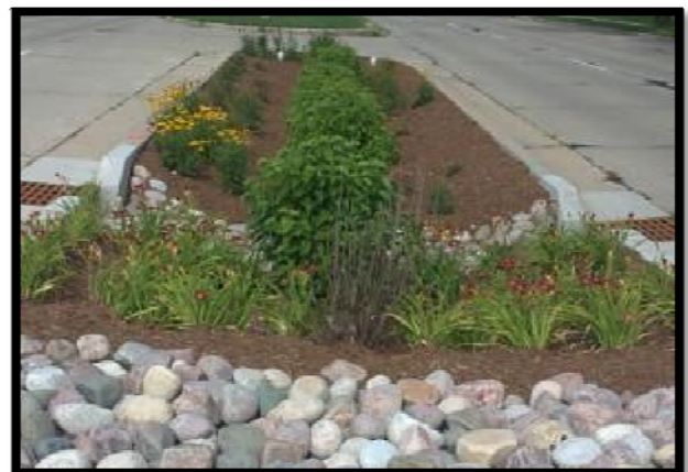
Median Bioretention Installation, Milwaukee, WI
