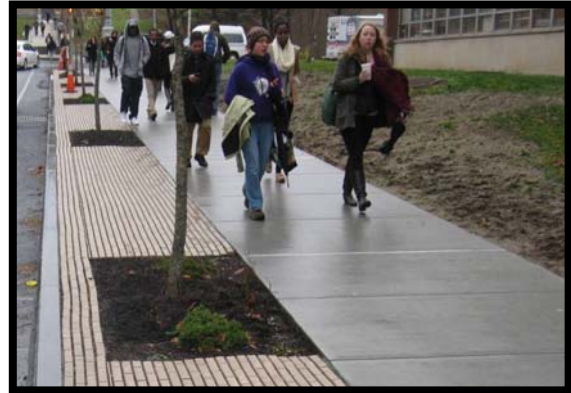
Tree Trench Installation, Syracuse, NY
