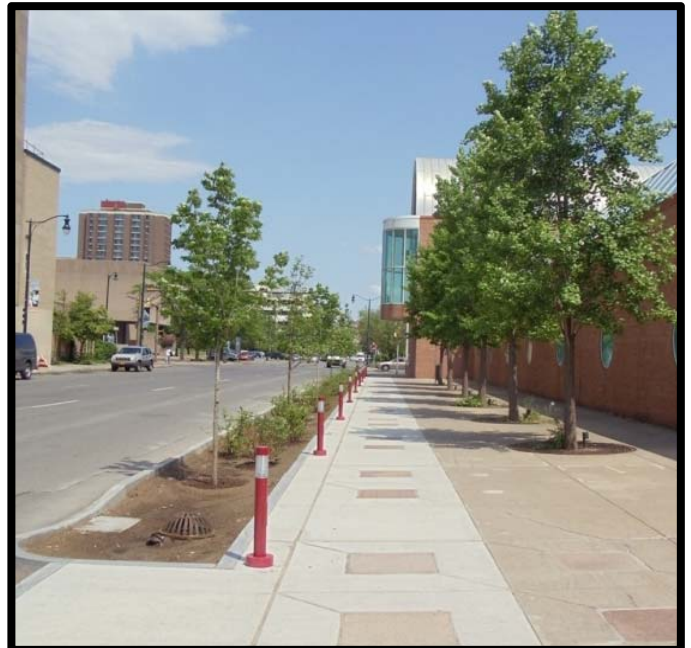
Urban Street After Curb Extension, Bioretention with Tree Planting and Overflow, Syracuse, NY
