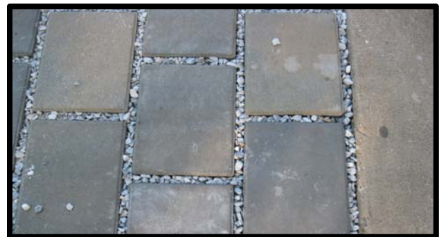
Close Up of Permeable Pavers
