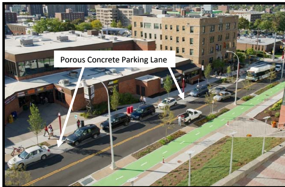
Porous Concrete Parking Lane, Syracuse, NY
