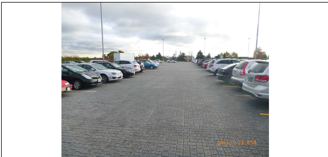
Fall 2013 – IMAX Permeable Pavement Parking Lot
