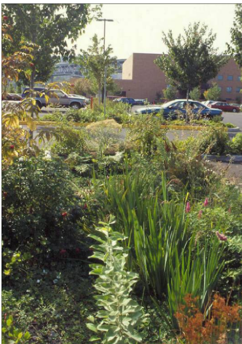
Figure 1: Vegetated Filter Strip
