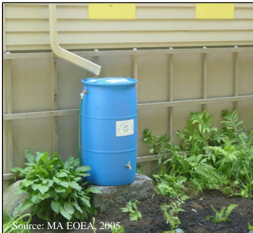
Figure 1. Residential rain barrel
