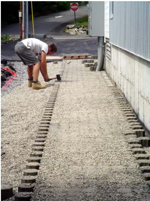
Figure 1. Installation of Permeable Pavers in a Driveway. Photo courtesy of Casco Bay Estuary Partnership.
