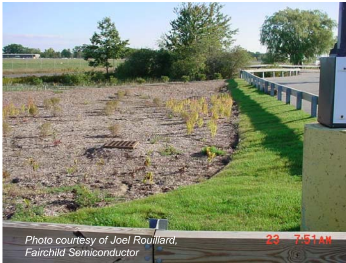
Figure 1: An Example of a Bioretention System (This system was recently planted and will fill in with vegetation over time.)
