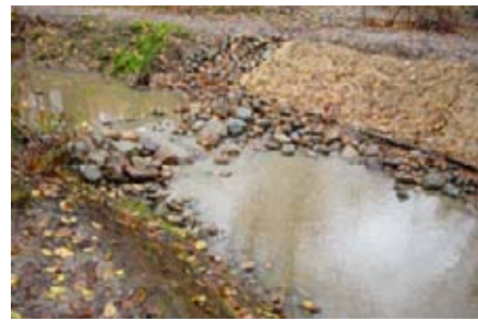
Many techniques are used to restore streams. Above, a newly installed rock riffle will slow stream flow and protect the creek from erosion. photo: http://waldendesign.net
