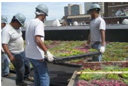
Workers install Hartford's first green roof on the Betty Ruth and Milton B. Hollander Foundation Center. photo: www.commonground.org
