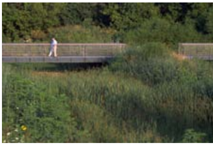
At Bear Grass Creek Preserve in Louisville, KY, the addition of constructed wetlands has reduced the number of floods in the adjacent creek. photo: WRT
