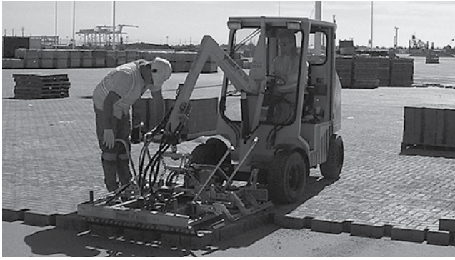
Figure 8. Mechanical installation equipment places concrete pavers rapidly.
