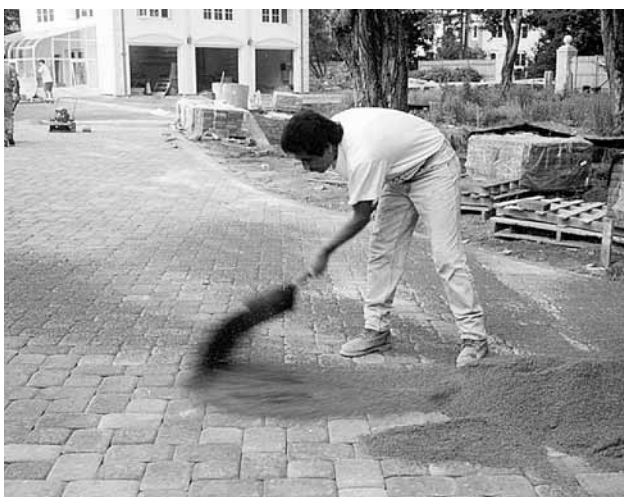
Figure 8. Spreading joint sand over the installed concrete pavers.
