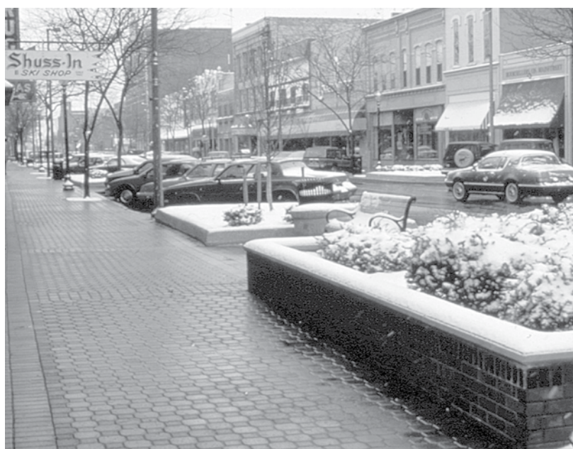
Figure 1. A snow melting system under concrete pavers in downtown Holland, Michigan has performed well since 1988.
