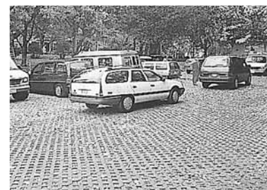
Figure 15. A parking lot with a dense-graded, crushed stone base.
