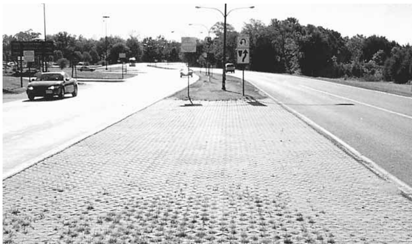
Figure 5. Roadway median crossover
