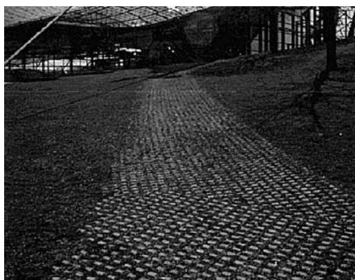
Figure 6. Service access lane
