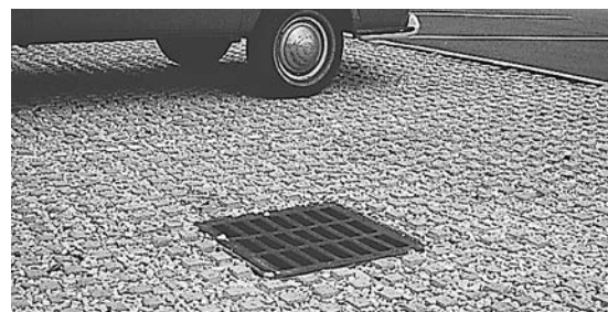
Figure 17. Concrete grids with aggregate in the openings
