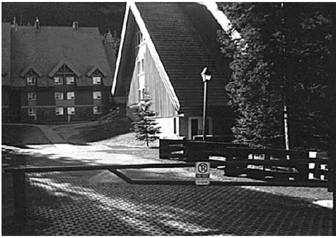
Figure 7. Emergency access lane for fire trucks
