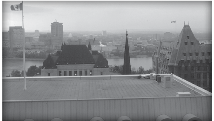
Figure 5. Light colored paving on low-slope roofs reflects light saving on air-conditioning costs while protecting the waterproofing.
