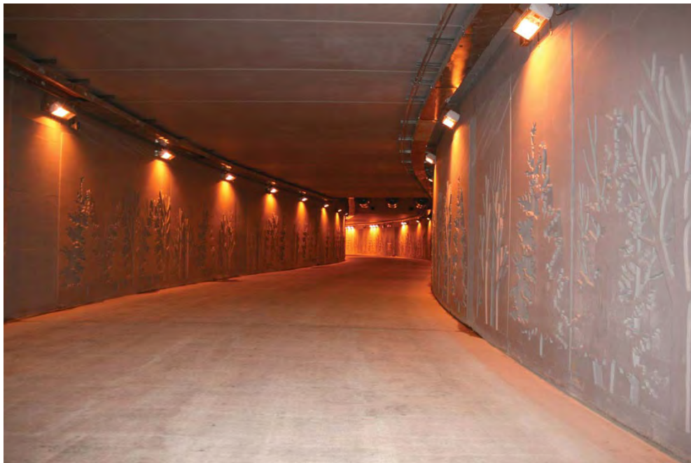
Figure AE-9.4: Seattle-to-Bremerton ferry tunnel in Bremerton, WA. Photo from the Washington State Department of Transportation.
