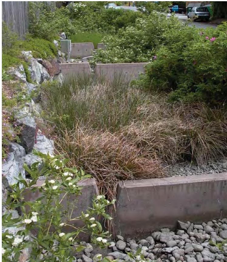
Figure EW-2.2: A bioswale with flow control weirs. (Photo by J. Anderson)
