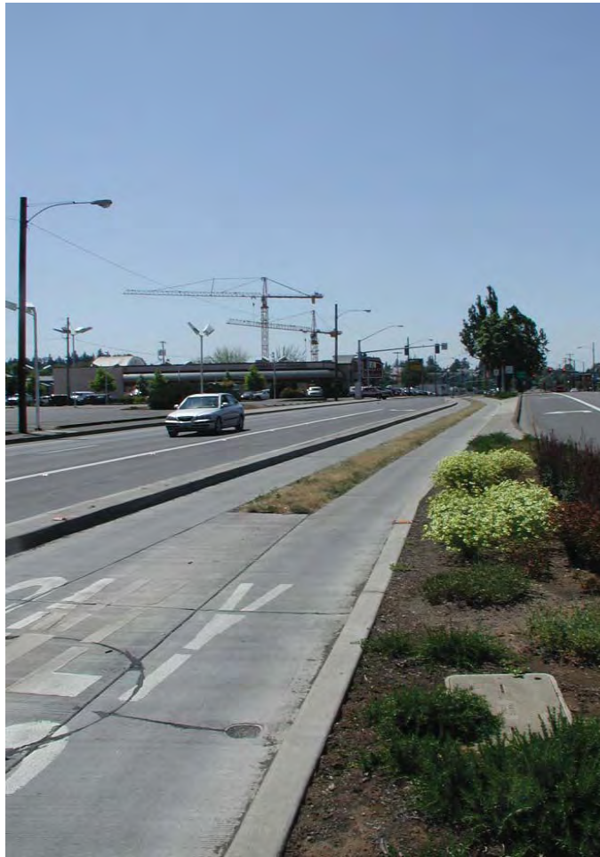
Figure AE-7.3: An at-grade transitway in Eugene, Oregon. 5 points. (Photo by K. Watkins)
