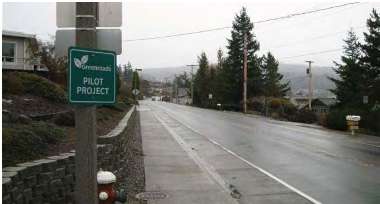
Figure I.1: Greenroads Pilot Project at Northshore Drive in Bellingham, Washington. Photo by Freeman Anthony, City of Bellingham Public Works
