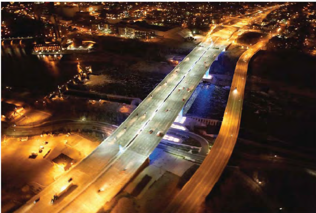
Figure MR-6.1: Aerial View of LED Lighting on I-35. Photo by Beta Lighting. http://www.ledwaystreetlights.com/Benefits/pdf/case-study/ledway-I-35W-CaseStudy.pdf
