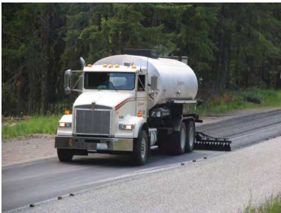
Figure MR-2.9: Chip seal asphalt emulsion application.
