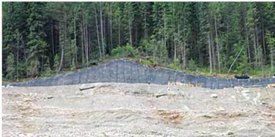
Figure MR-3.2: Tecco® high-strength steel mesh used for slope reinforcement. (BCMOT, 2010)
