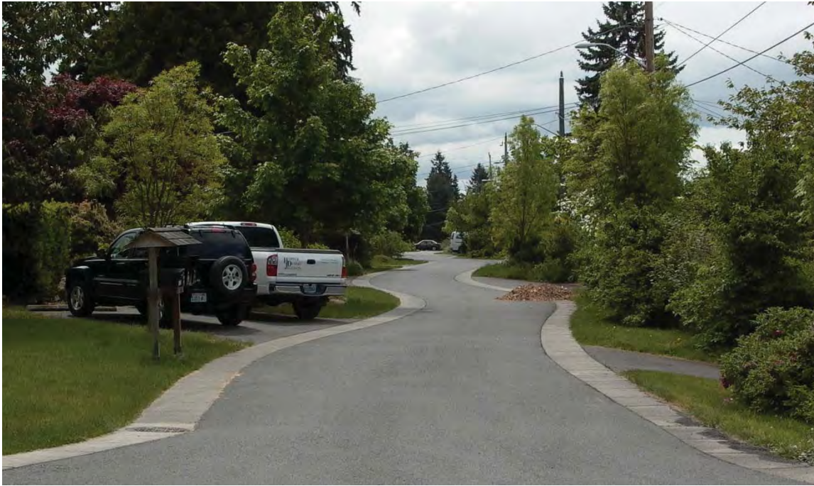
Figure PR-8.2: This street was designed to be narrower in order to produce a traffic calming effect for this residential area. (Photo by J. Anderson)
