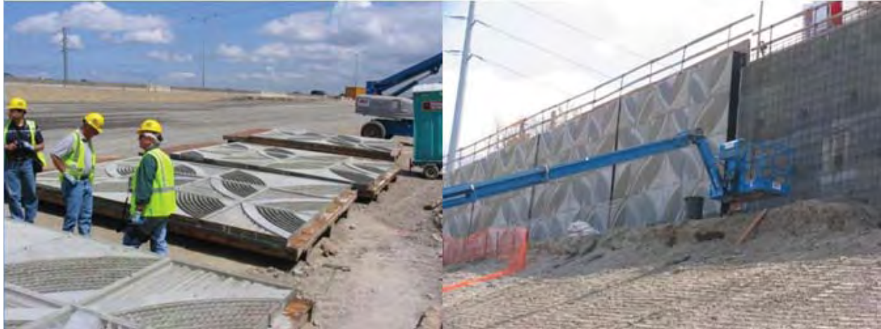
Figure AE-9.3: Art incorporated into the fascia for an I-5 freeway wall associated with an expansion project on I-5 near its intersection with SR 16 in Tacoma, WA.
