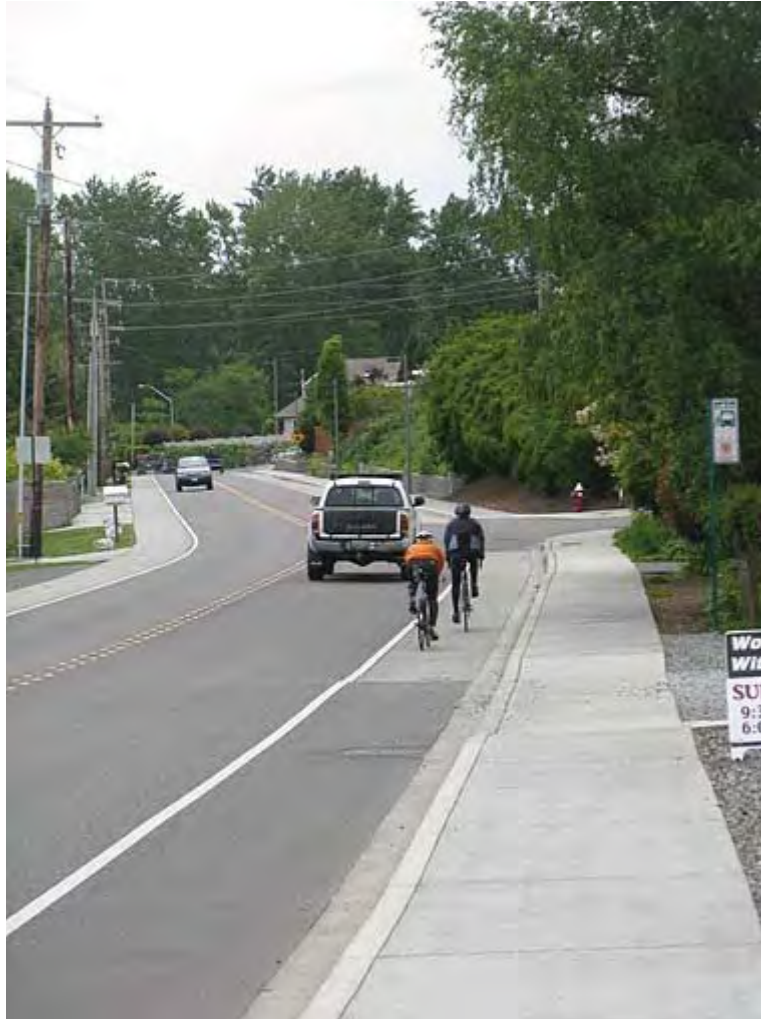
Figure 1: Northshore Drive in Bellingham, Washington. Cyclists using permeable pavement bikelanes adjacent to permeable sidewalk. Photo by C.Weiland
