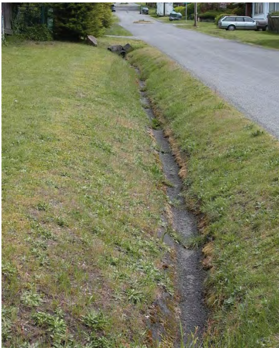
Figure PR-8.3: A conventional asphalt lined channel near SEA Street. (Photo by J. Anderson)
