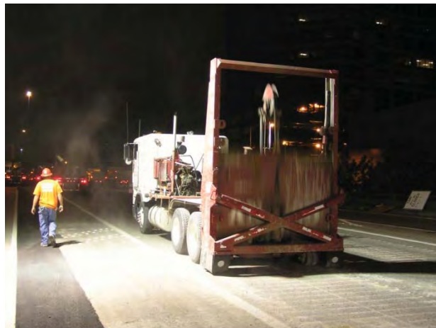
Figure MR-2.18: Guillotine breaker used for crack-and-seat.
