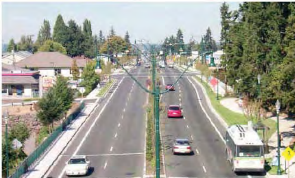
Figure AE-6.5 - Bridgeport Way After Construction (Context Sensitive Solutions, 2005)
