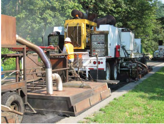
Figure MR-2.13: HIR heating equipment.
