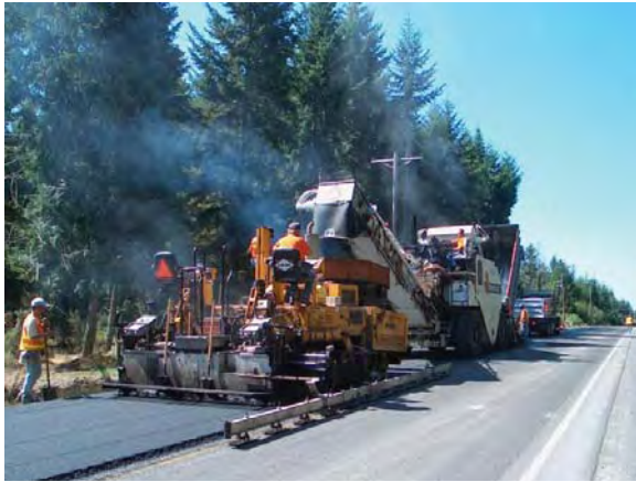
Figure MR-2.11: 1.8-inch overlay.
