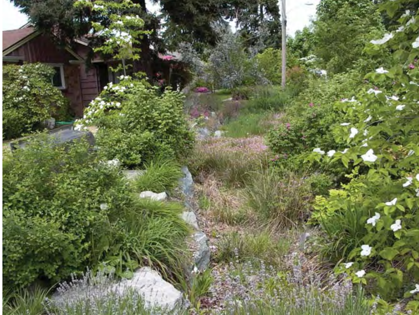
Figure EW-3.2: A well-established vegetated swale (“bioswale”) that uses compost amended soil and no flow control devices or structures. Residential street to right. Seattle, WA. (Photo by J. Anderson)
