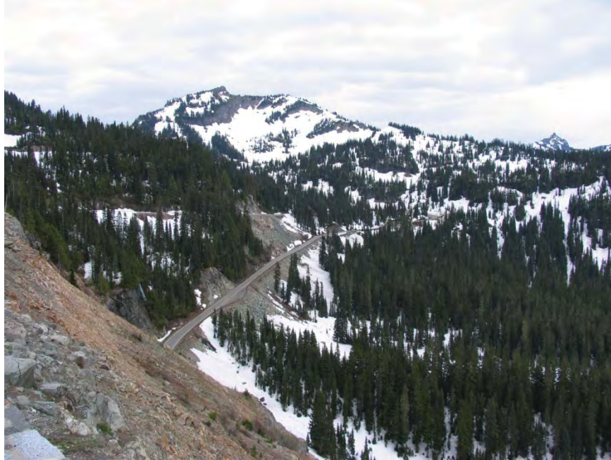
Figure AE-8.4: Scenic pull out (slightly left and lower from center) on SR 410 in Mt. Rainier National Park.
