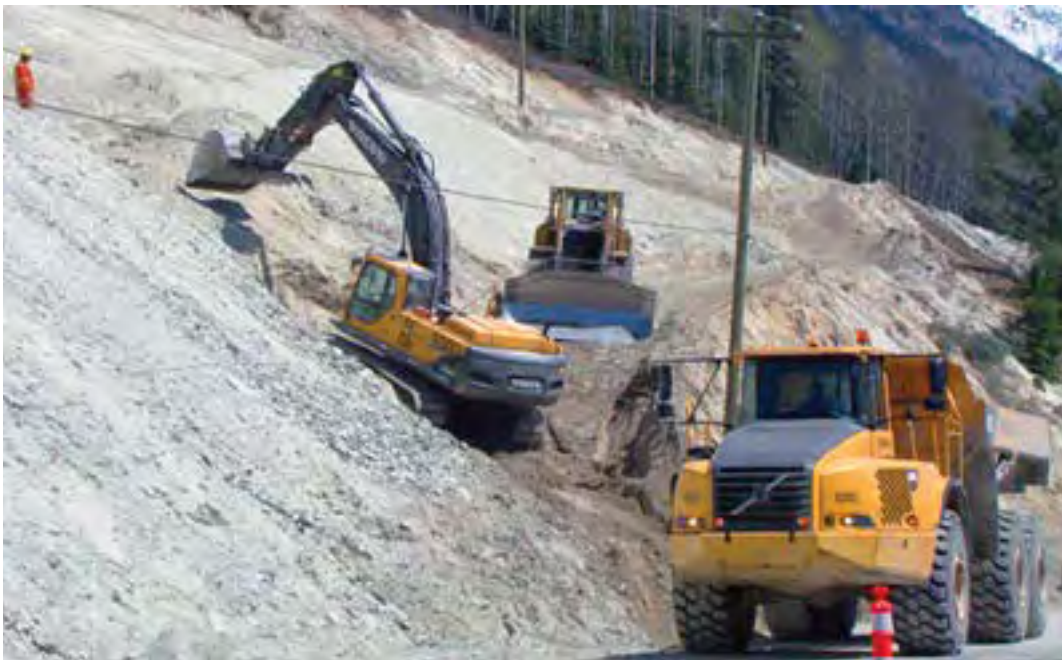
Figure MR-3.5: Phase 3 earthwork on east side of highway (BCMOT, 2010)
