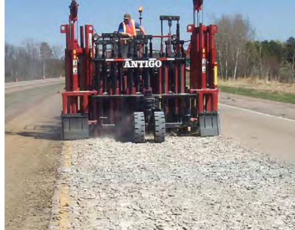
Figure MR-2.20: Antigo multi-head breaker (photo from Antigo Construction, Inc.).
