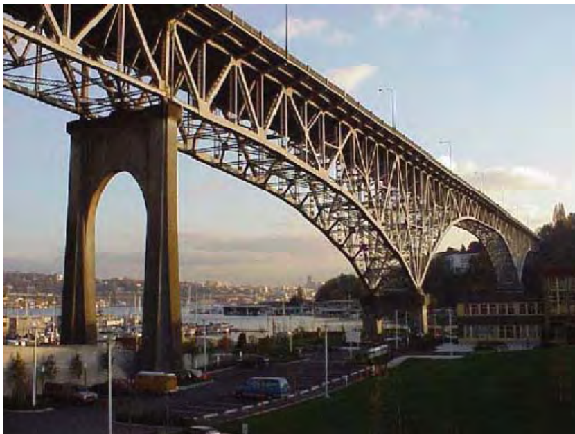
Figure MR-2.5: Aurora Bridge, Seattle, WA (Photo Courtesy of WSDOT)
