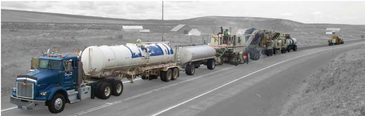
Figure MR-2.15: CIR process train (photo from the Washington State Department of Transportation).
