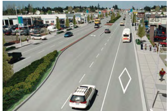
Figure AE-3.2: Aerial view of Aurora Avenue and BRT. Photo by CH2M Hill.
