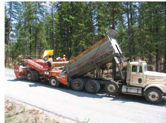
Figure MR-2.10: Chip seal aggregate application.
