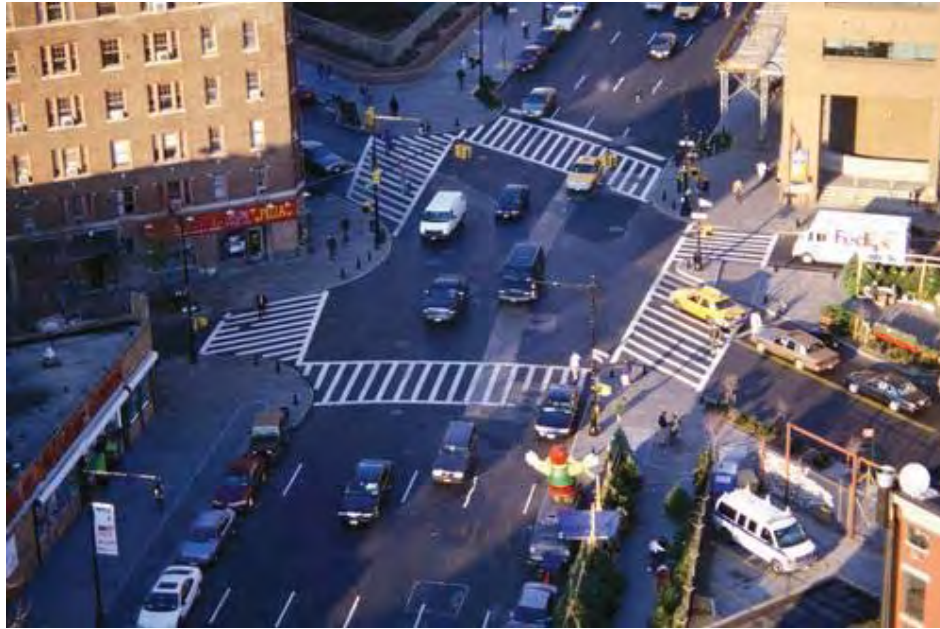
Figure AE-5.2 - Mulry Square After Construction (Context Sensitive Solutions, 2005)
