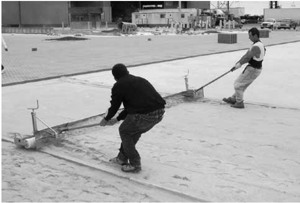
Figure 4. A two-man hand pulled screed
