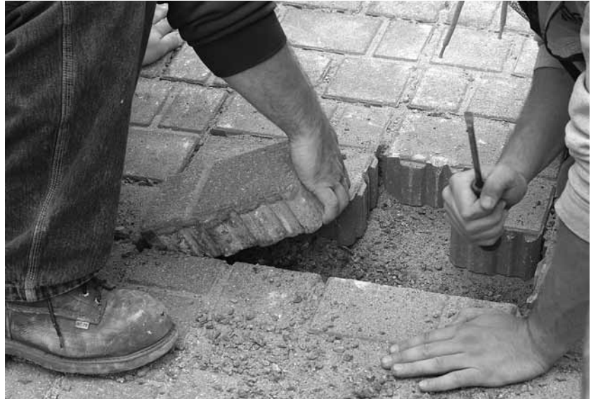
Figure 7. Pulling out a paver by the short end provides greater leverage and makes extraction easier.
