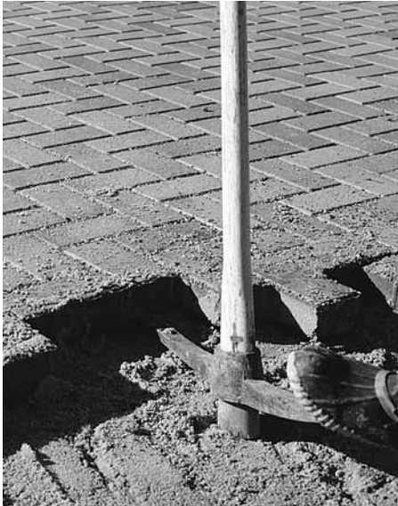
Figure 6. Prying out the remaining pavers
