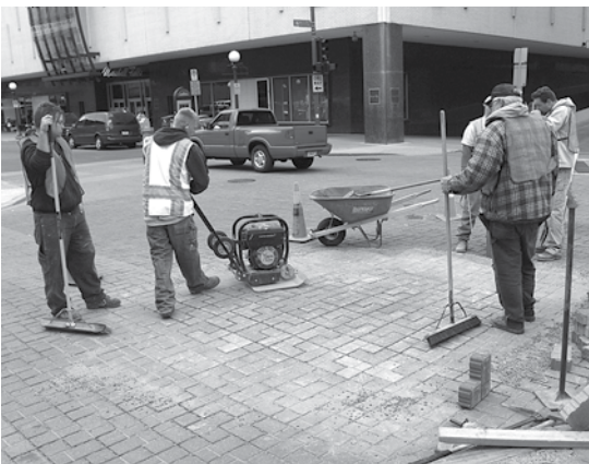
Figure 15 and 16. Reinstated pavers leave no ugly patches nor do they weaken the pavement.
